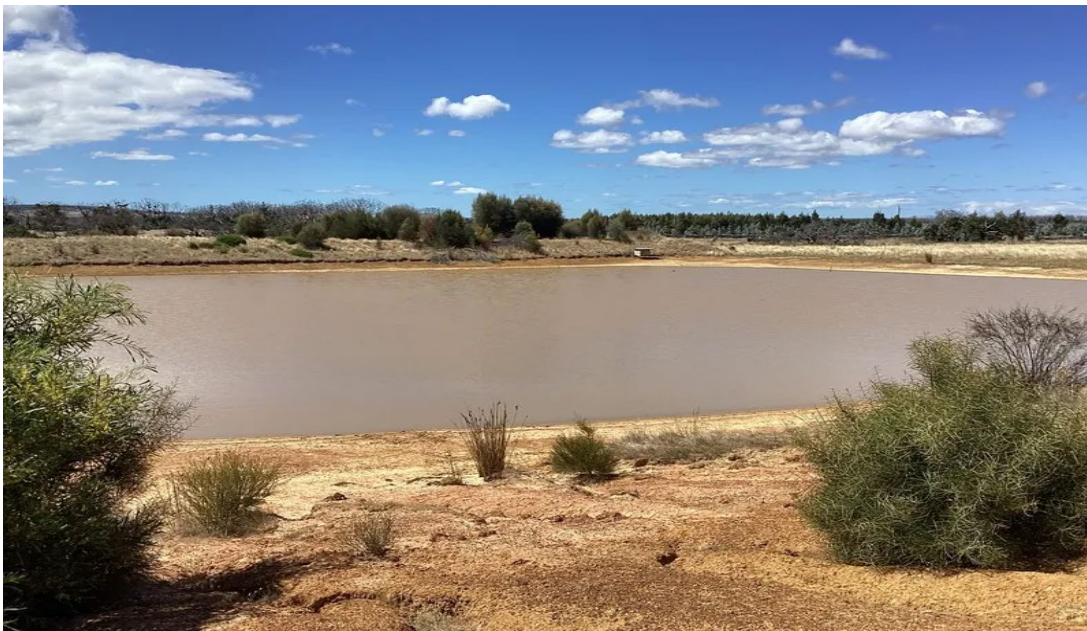
Water Infrastructure – Lot 58 South Coast Road, Karrata
