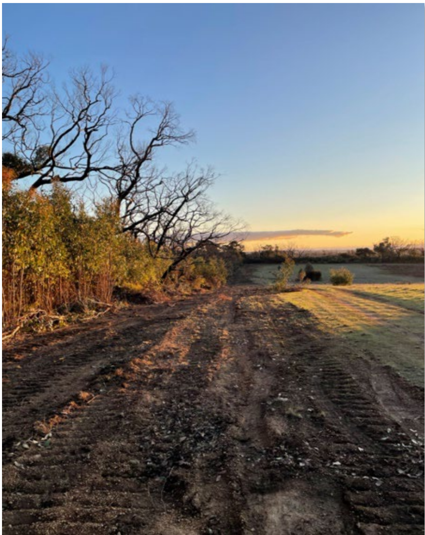
Line ready to be fenced at Morlands
